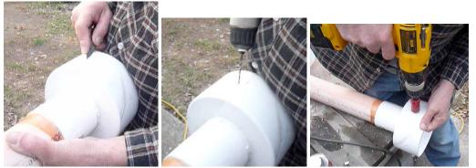
Drill a 1" hole in the side of the base, to allow the hose to come out. A slot would work too, if you don't have a hole saw.
